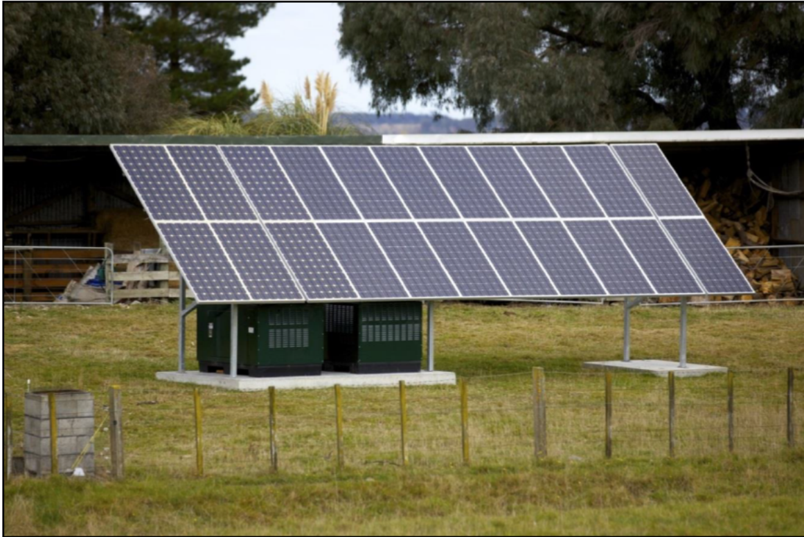
Figure 3: Example of SPS installation - Source: Powerco (New Zealand)
