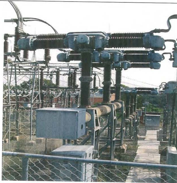
Figure 1 – Air-Blast Circuit Breaker
