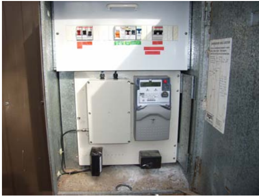
Single-phase residential smart meter with external modem power supply.
