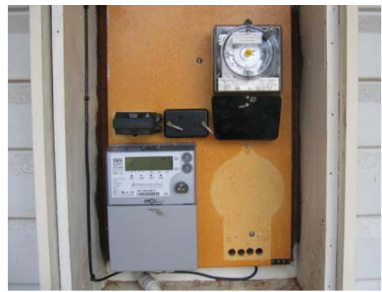
Single-phase smart meter with external timeswitch.
