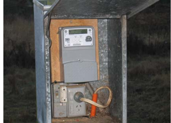
Single-phase smart meter – rural dam pump.
