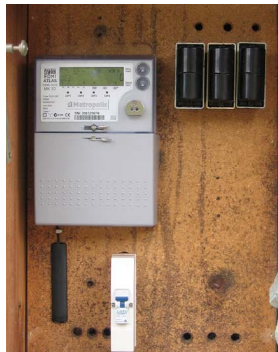
Three-phase residential smart meter.
