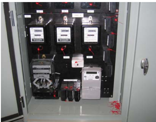
Single-phase residential smart meter – block of units.
