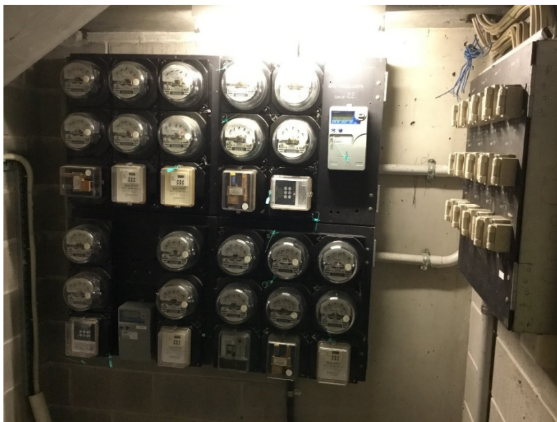
Example 3. - The following picture shows a more complex board services many NMI' with a single Isolation point.
