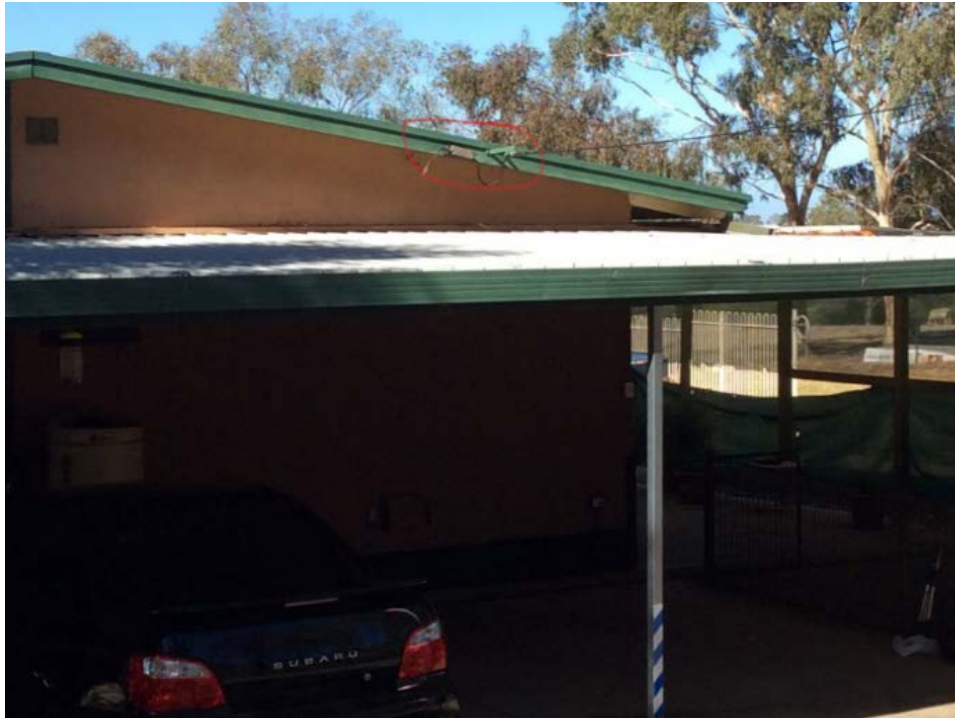
Example 6. - Unable to access fuse. This following example shows the isolation point obscured by vegetation. Customer would be required to resolve this issue before metering work can be performed.
