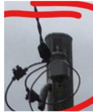
Example 8. - Unable to access fuse - In the below example porcelain bell housing fitted are difficult to operate and are subject to total failure when pulled with a fuse stick. Should they fail a simple job becomes much more complex with a customer left off supply.
