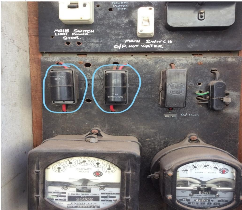
Example 5. - Unable to access fuse – this is where the point of isolation exists but is no longer accessible. In this example a carport has been constructed that limits safe access to the service fuse. This will be in contravention of the customer's connection agreement. It is likely a DB would require the customer to resolve this issue.
